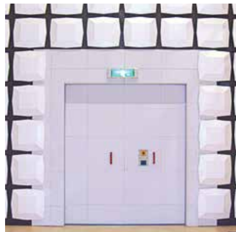
Inside View of Semi-Auto Sliding Door
